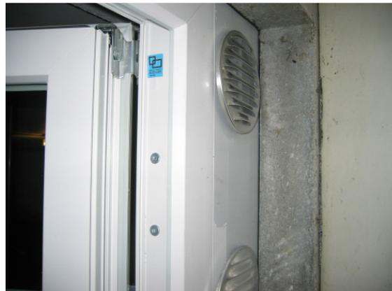
Montage des Abluftventilators
